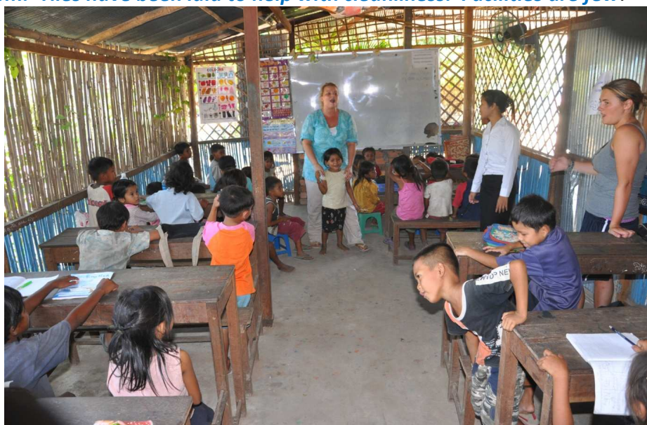
Current classroom with bamboo walls and concrete floor – a problem in wet weather
